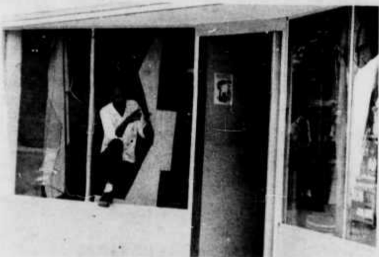
COFO Headquarters after window smashing.
