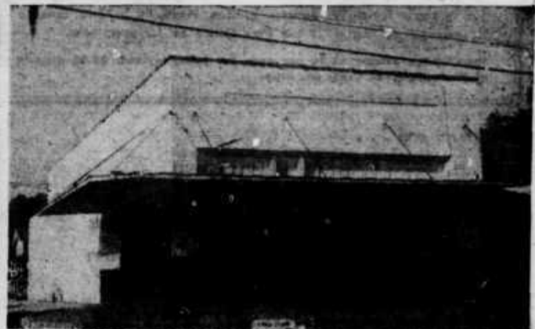
JORDAN SUPERMARKET —The store looks mighty dark under that awning in front, but it's not because our picture is under-exposed. The reason is that there is nothing inside the store. Jordan's on Lynch St. was cleaned out by the boycott.
